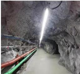
Figure 3: Underground passageway with compressed air and water pipe (red and green) with electric overhead lighting.
